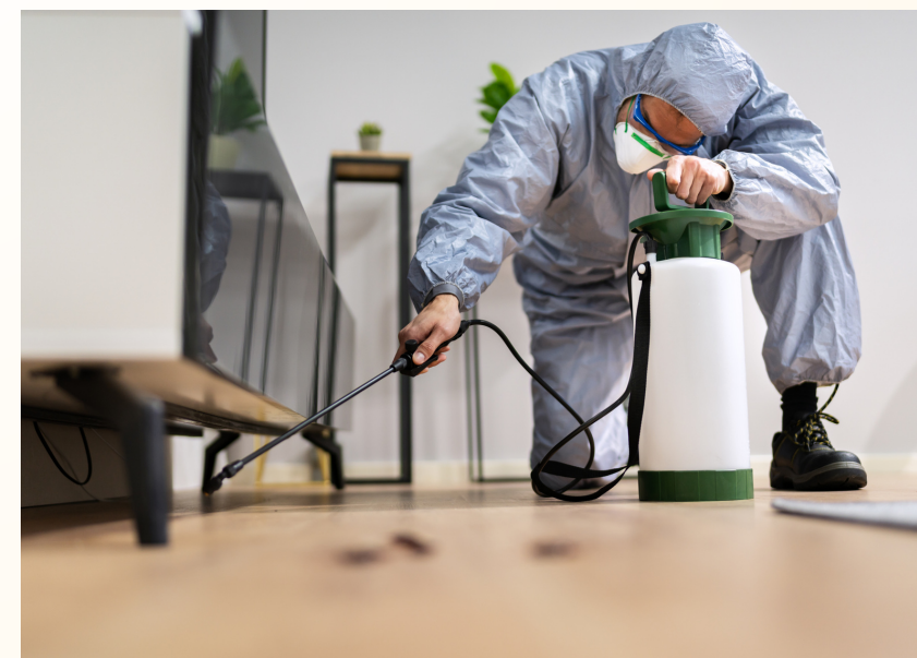
Anti Termite Treatment
